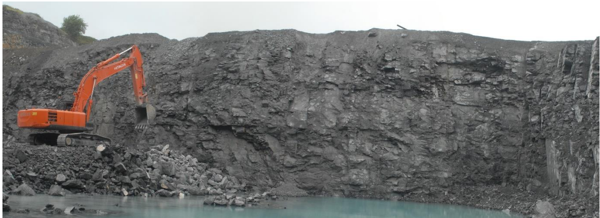
Active face looking NE from IM 52088 13158. Bedding and joint surfaces are partially obscured by dust.
